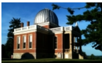
The main observatory building
